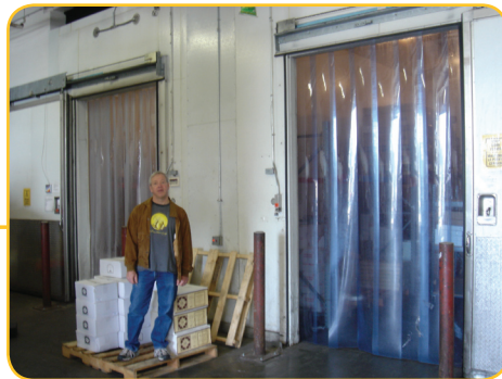
Refrigeration Strip Curtains at NORTHWEST CHEESE DISTRIBUTORS 1012 Revere St.
